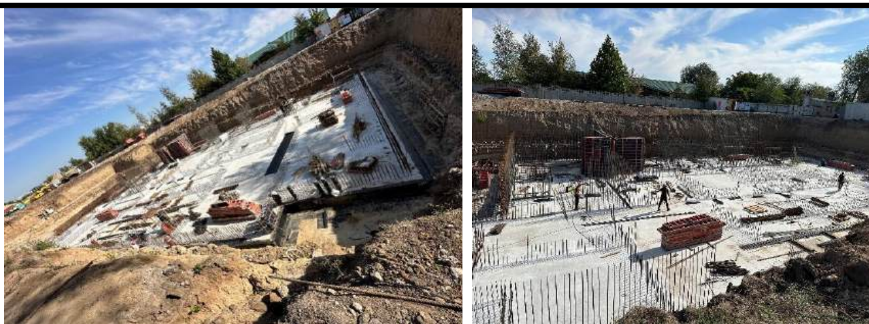
Figure 2. Construction of a bomb shelter in the Dnipropetrovsk region
