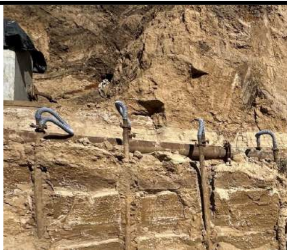
Figure 4. Drainage of the construction pit with needle filters: 1 – construction pit; 2 - needle filters.
